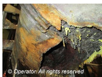
Sulphur leak from the heat exchanger
