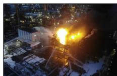
A fire occurred at a distillation unit in a refinery. Between 300 and 600 m<sup>3</sup> of flammable substances were involved. Approximately 2,500 m<sup>2</sup> was impacted. Fortunately, no injuries were caused by this accident. But there are still many lessons to be learnt from analysing its root causes. The report explores several of them. The origin of the initial leak? Late detection of alarms? Coordination between the internal firefighters and the operator?
