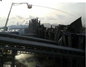
unit (with biofilters spanning 3,000 m<sup>2</sup>). In less than an hour, the fire had reached another sorting zone (5,000 m<sup>2</sup> of floor area containing plastics). The outbreak continued its course via conveyor belts crossing the firewalls and the glued-laminated wood frame covering these walls; burning timber fell to the ground, igniting 2 household waste pits (27,000 m<sup>3</sup> over a 20-m thickness) around 6:30 am.
