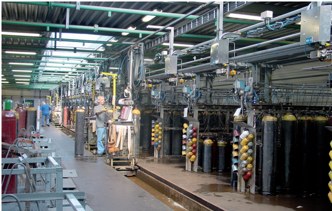
Automated industrial gas bottling chain (Emerson Process, ARR)
