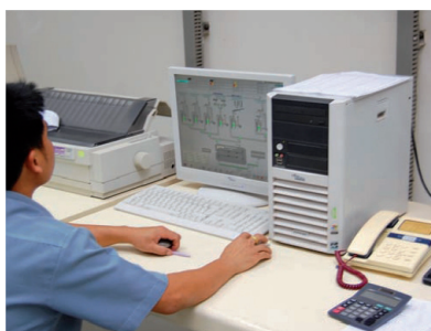
Programmation d'un automate (source : Control Engineering Asia)
