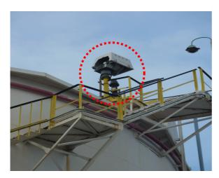
Figure 5: View of the radar device on tank T 495 (source: DREAL-ALSACE)
