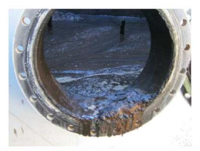
Fig. 12: Solid / paste residues collected from the exit nozzle (source: operator)
