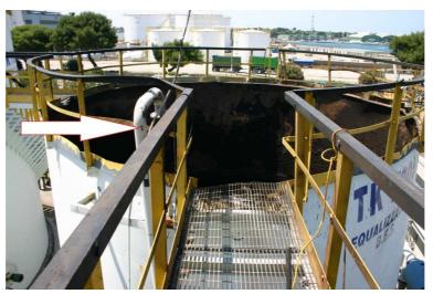
Fig. 5: Pulled-off sparger line on the TKX viewed from the walkway (source: ARPA Puglia)
