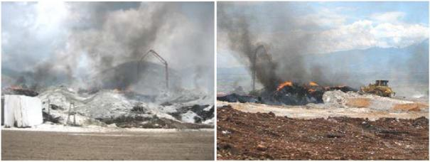
Concrete being pumped on the burning pile. Burning pile being covered with soil. (photos taken by the Environmental Inspectorate)
