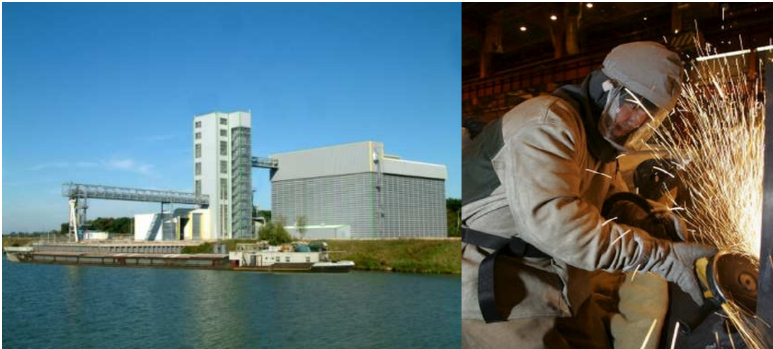
Photo COOP de FRANCE
