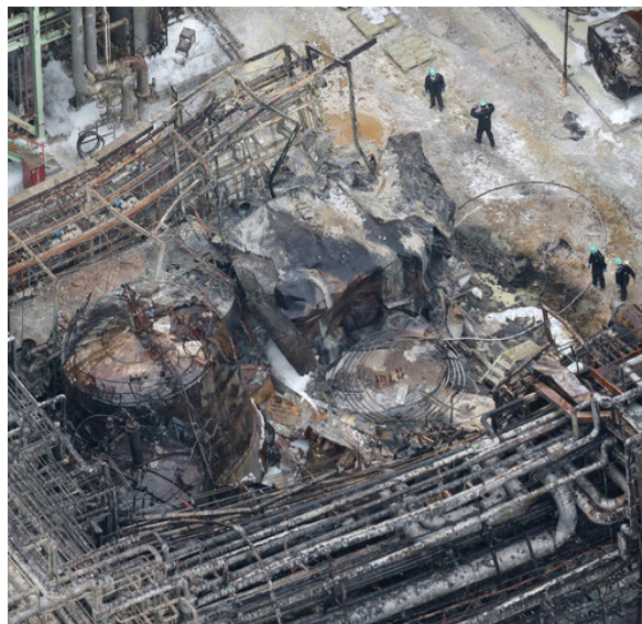
Fig. 11: View of damage after the BLEVE explosion (Source: operator)
