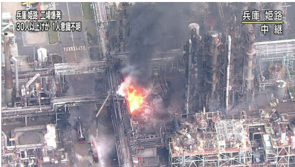
Fig. 9: View of the damaged unit after the BLEVE-type explosion (Source: Japanese television report)
