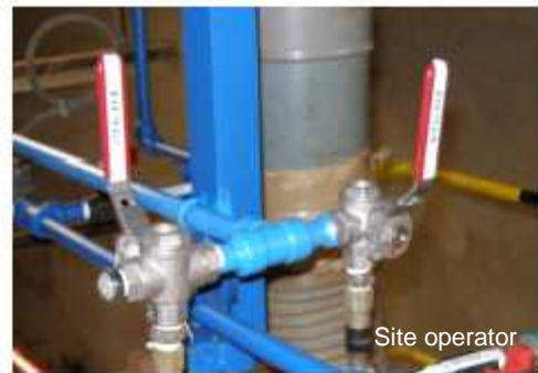
Installation of 3-way valves
