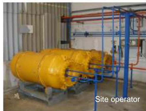
Installation of "liquid traps" in both high-pressure circuits
