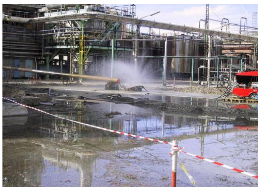
Dilution of NH 3 by water curtains
