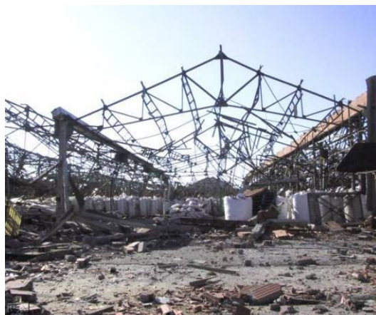
Warehouse destroyed by the blast
