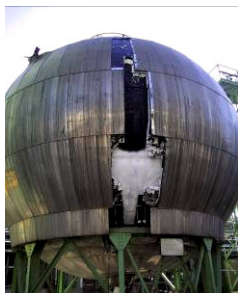
Superficial damages suffered by a NH 3 tank
