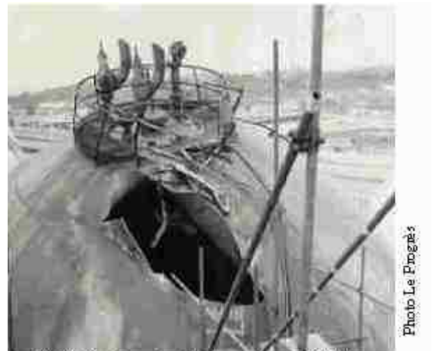
Figure 10 – Opening in butane sphere T 61441
