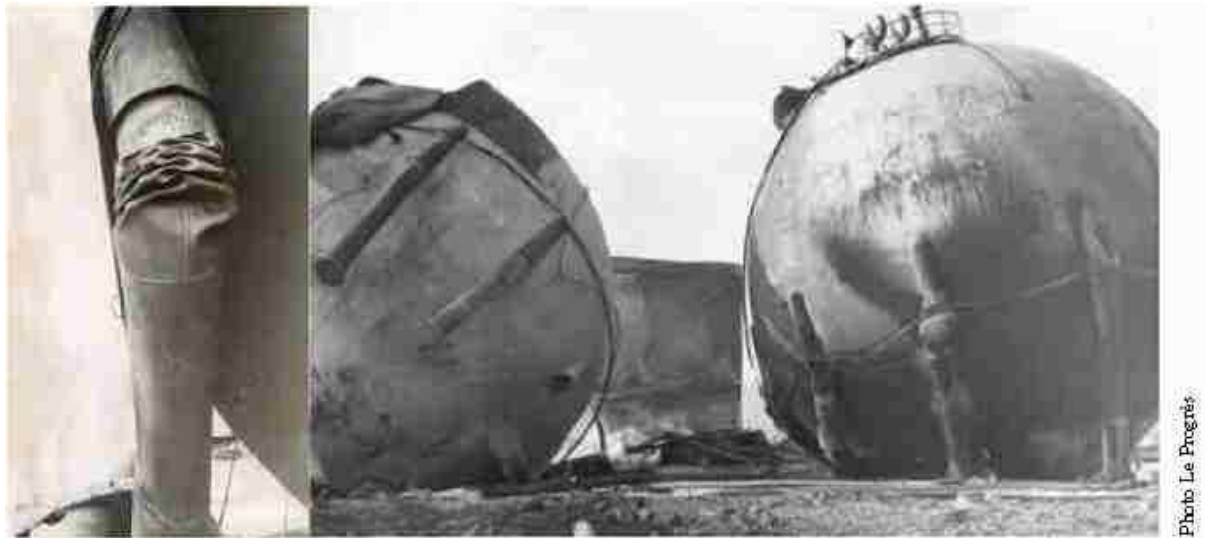
Figure 14 - Illustration of the general condition of the spheres damaged in the explosions.
