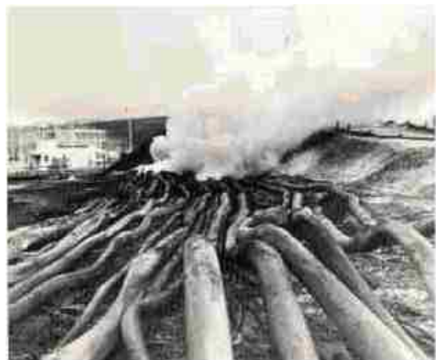
Figure 12 – Pipe damage
