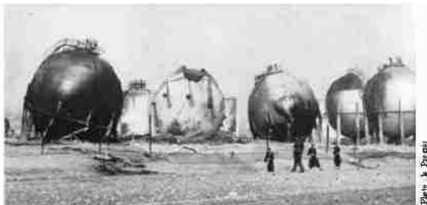
Figure 5 - General condition of the LPG spheres after the accident
