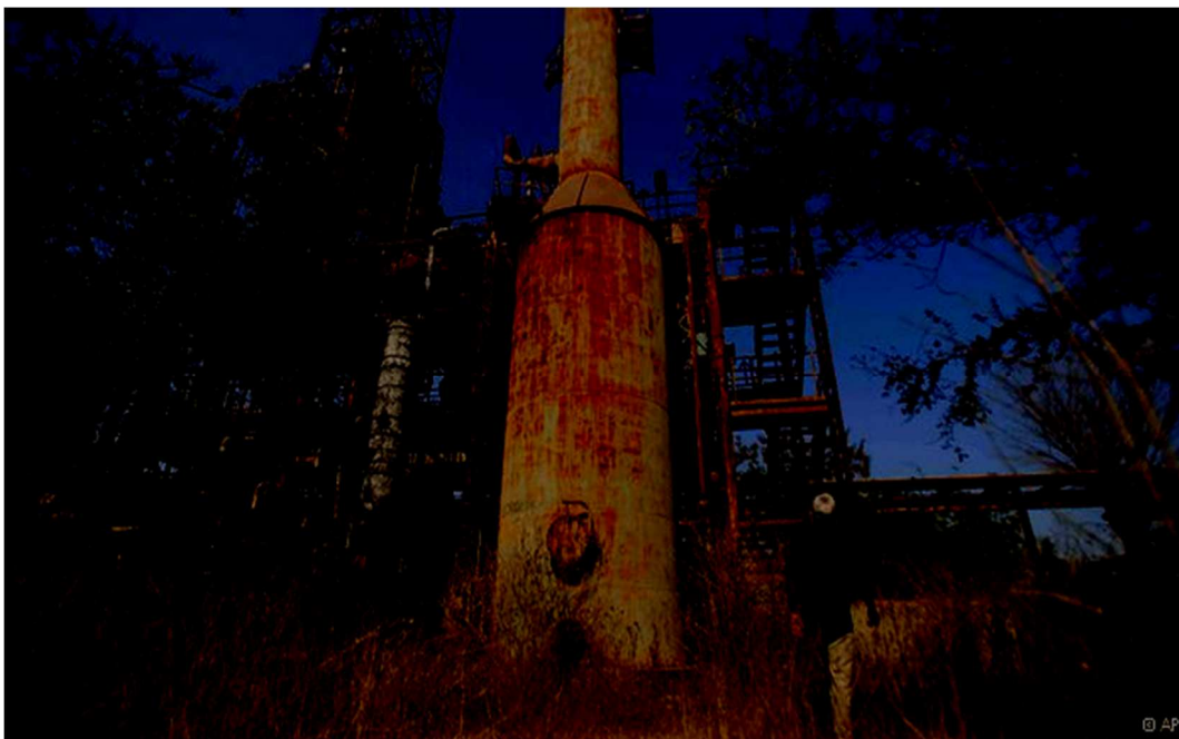
Remains of the Bhopal installations today [12]
