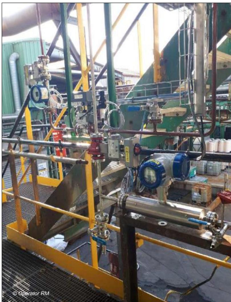
The operator also made technical modifications to their facility. They moved the combustible fluid pipe / valve / flow meter groups away from the after-burner wall.
