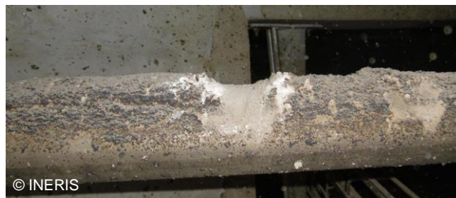
Example of dust accumulation in the sub-cell gallery
