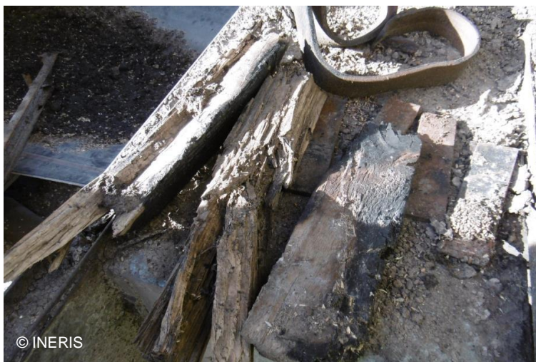
Pieces of wood trapped in the hopper
