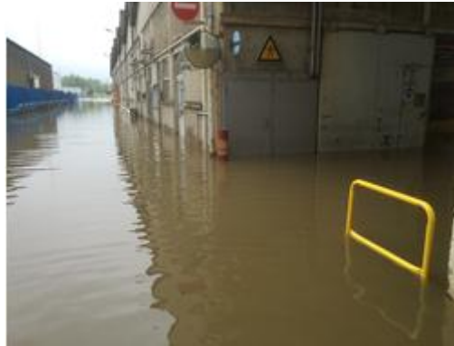
The flooded installation - source: operator
