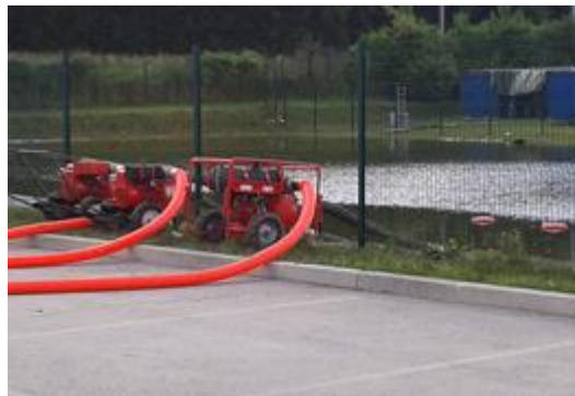
Water pumping operations - source: operator
