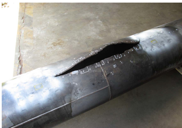
Copyright: Pipeline operator
