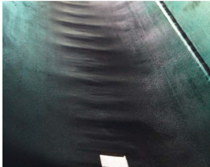
Copyright: Pipeline operator
