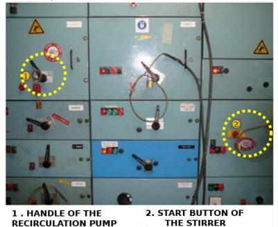
Fig. 11: View of the control board for the process implicated in the accident (Preventique Group)
