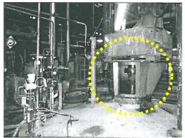
Fig. 12: Stirrer motor and shaft visible on the upper part of adjustment tank T76 (plant operator)
