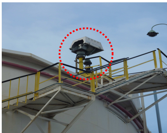
Figure 5: View of the radar device on tank T 495 (source: DREAL-ALSACE)
