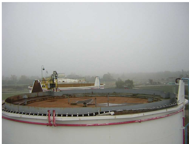
Figure 4: View of the tank's floating roof after the overflow (source: Site operator)
