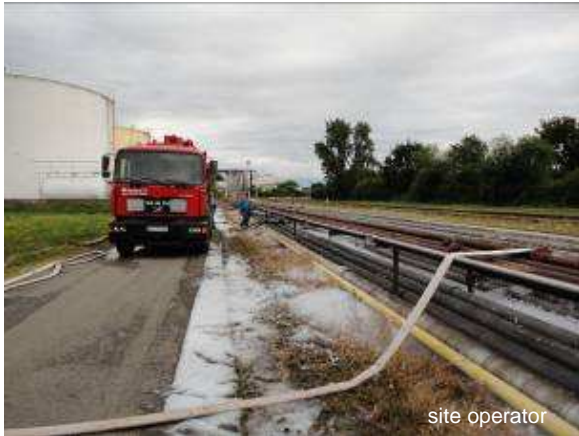
Place of the accident the day after
