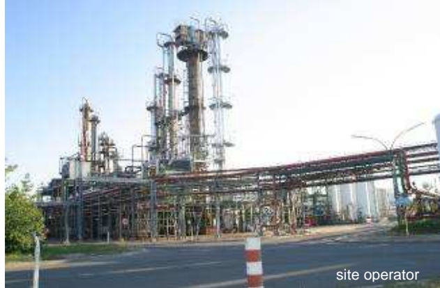
Production facilities and pipes rack
