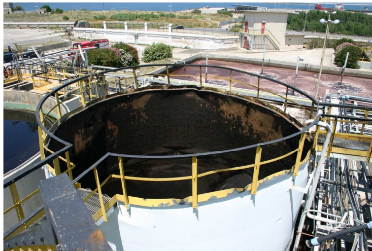
Fig. 7: Exploded TKX (source: ARPA Puglia)
