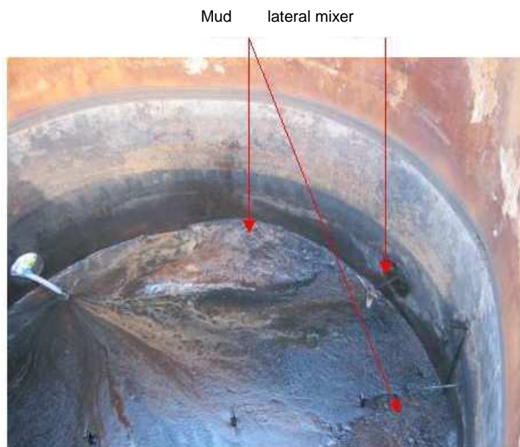
Fig. 11: TKX after emptying in December 2000 - solid residues collected from the bottom (source: operator)
