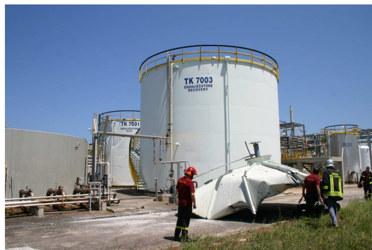
Fig. 8: Projected roof at the foot of the TKX (source: ARPA Puglia)
