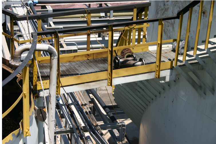
Fig. 6: Walkway between TKX and TKY (source: ARPA Puglia)
