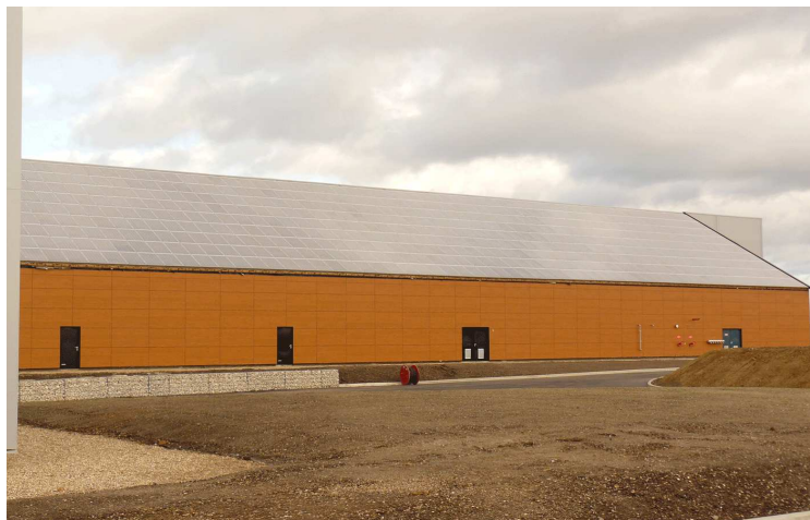
The industrial building and its roof composed of photovoltaic panels, prior to the accident - DR
