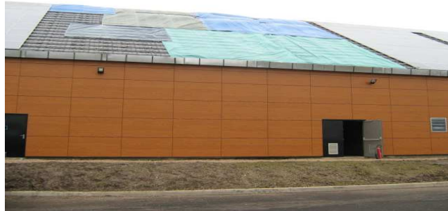
Covering of the damaged roof with a tarp (source: DREAL)
