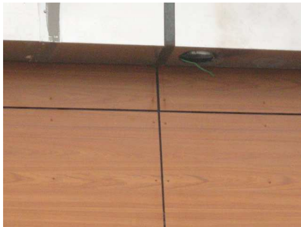
Location of the exact spot where works took place (source: DREAL)
