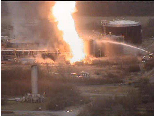
Figure 4: Ethylene jet flame from the broken bypass of the gate valve; gas pressure: 83 bars. Half an hour later the nearest acrylonitrile tank caught fire.
