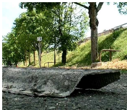
Debris found in Z4 (Source: site operator)
