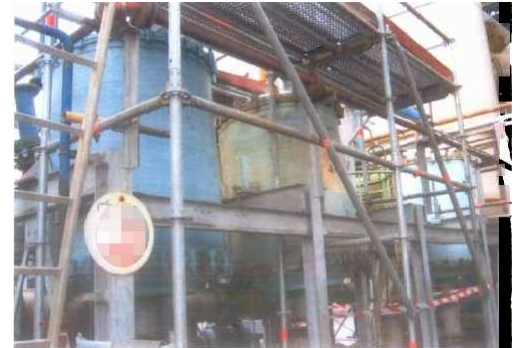
Replacement of the exchanger
