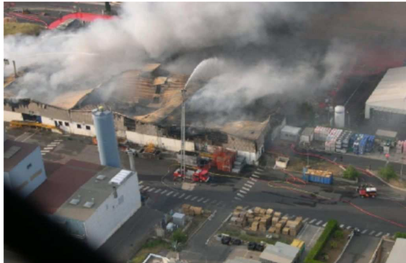
Spread of the fire to several buildings
