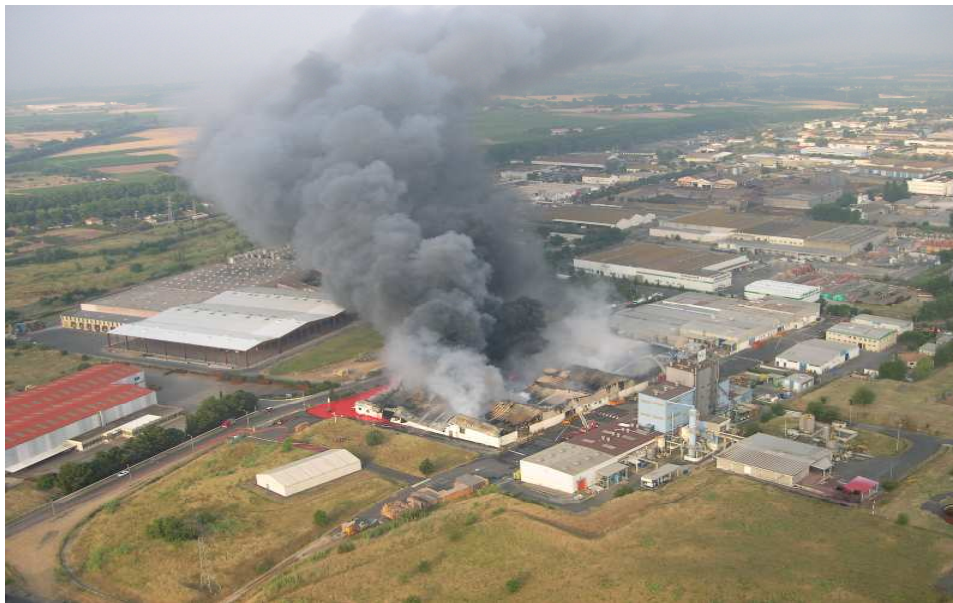
Plume of smoke rising above the site
