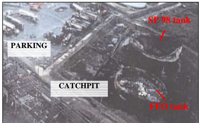
Aerial view of the tank farm
