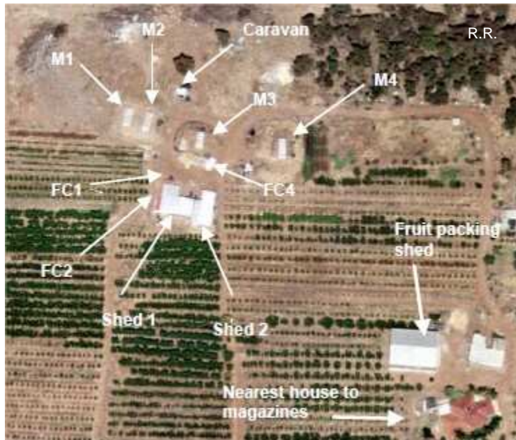
View of the storage facility - FC3 is located inside shed n2 [1]
