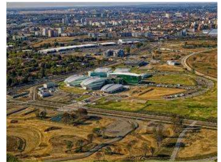
The cancerology center under construction (source : Oncopôle Toulouse )
