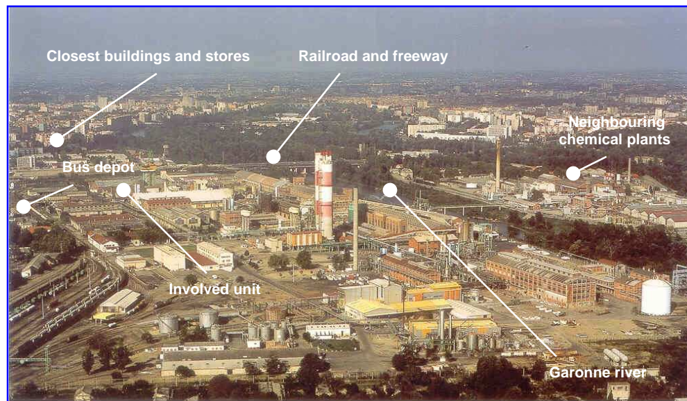
View of the plant before the accident (source : Grande Paroisse)
