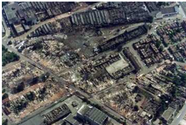
Aerial view of the site following the accident [3]
