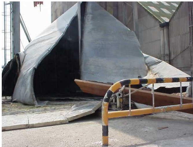
Destroyed reservoir (Source DRIRE)
