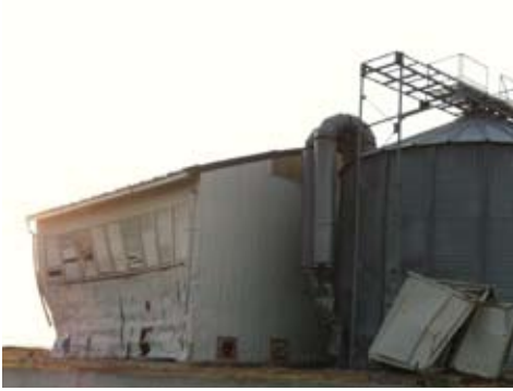
Above: exterior and interior photos of a grain silo damaged by the tsunami and its debris near Natori (Source : DGPR), Right: liquefaction of the dock of a grain silo in the Port of Kashima (source: METI)
