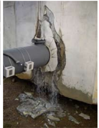
Damaged pipe of a settling basin (amateur photo)
