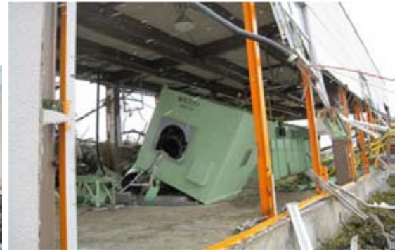
External damage: aeration tanks, pipes, treatment equipment (Source : Miyagi Prefecture - JWSA)
