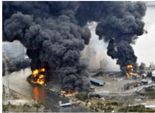
View of the road/rail loading station during the fire (amateur photos). A leak on a petrol pipe is the likely cause of the hydrocarbon vapour cloud, which ignited
