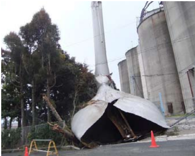
Cement plant in Hitachi; water storage tank ripped open by the earthquake (amateur photo)
