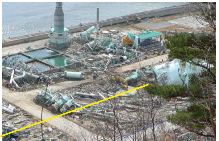
Above: Outdoor water and fuel-oil storage tanks swept away by the tsunami. Left: Surface facilities of the Kuji strategic national reserve. The underground fuel storage tanks were unscathed but seawater had to be pumped out. (amateur photo)
