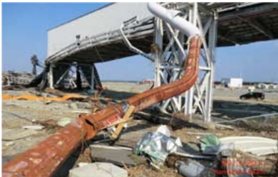
Port coal conveyor damaged by the tsunami at the Sinchi-Soma plant (Source: SPA Risk)
