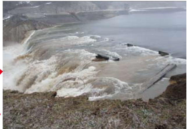
Breach of the main dam on March 11th, 2011 at 15.11 (Source : M. YOSHIZAWA)
