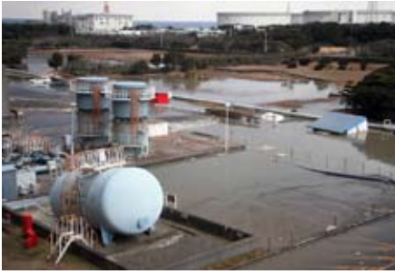
Soil liquefaction outside the Kashima plant (Source: TEPCO)
