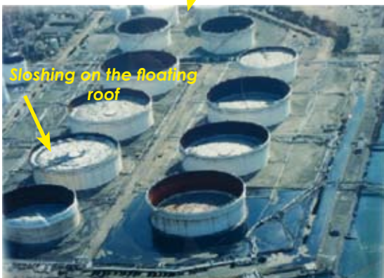
Sloshing on the floating roof Although they were empty, the crude-oil storage tanks (2 million m 3 ) stayed in place during the 3.5 m tsunami. The pipes, however, gave way after being pushed up by the incoming water. (Source : NRFID)
