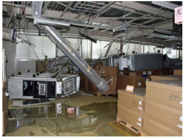
Collapsed AC duct and water on the floor of the storage area (Source : Fujitsu)
