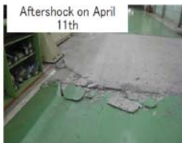
Widening of the floor cracks between March 11 th and the aftershocks of April 11 th 2011 (Source : Nissan)
