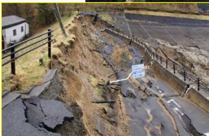
View of the slide in the auxiliary saddle dam, probably triggered the rapid emptying of the reservoir (Source : GEER / L.F HARDER)
