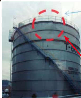
Warping at the base and top of the shell of a 5,000 m 3 storage tank in the Niigata oil terminal on March 11 th (Source : NRFID)
