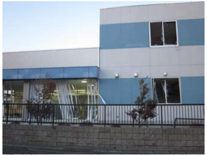
Effect of the hydrogen explosion on the KUREHA plant of Iwaki (amateur photo)
