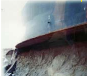
Soil erosion, as much as 3 m deep in places, caused by the tsunami around the large storage tanks (Source : JX)
