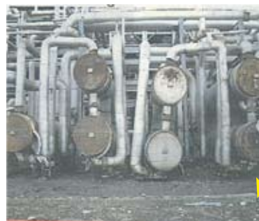
Collapsed foundations of the heat exchangers (Source : JX)
