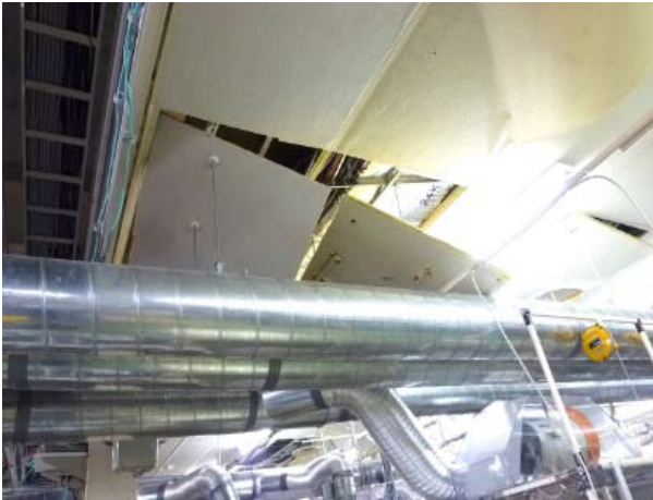
Damage to the suspended ceilings on the second floor of the main building (Source : Fujitsu)
