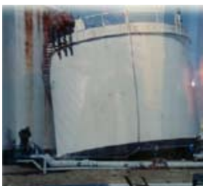
Small empty storage tank (3,000 m 3 ) pushed off its foundation by the tsunami (Source : NRFID)
