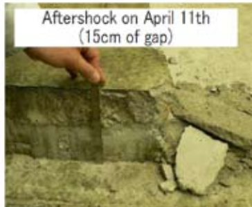
Excavation of the floor prior to repairs (Source : Nissan)
