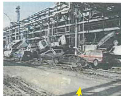
Below: Vehicles in the racks of the propylene fluid catalytic cracking [FCC] unit ( Source : JX)
