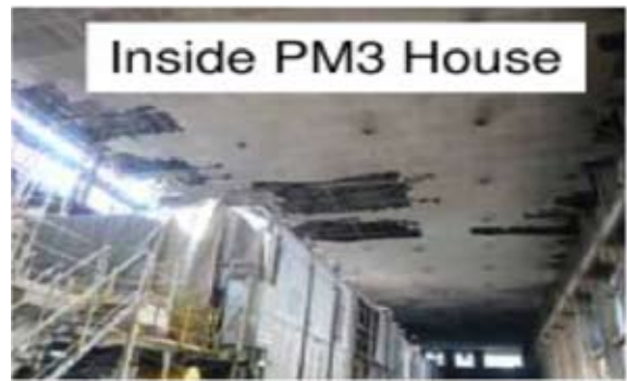
Iwanuma paper mill in Soma: seismic damage sustained by the building housing the paper calenders (Source: Nippon Paper)
