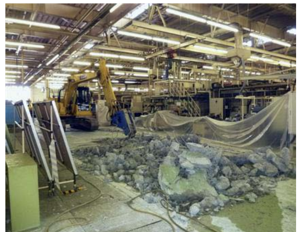
Excavation of the floor prior to repairs (Source : Nissan)
