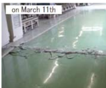
Widening of the floor cracks between March 11 th and the aftershocks of April 11 th 2011 (Source : Nissan)
