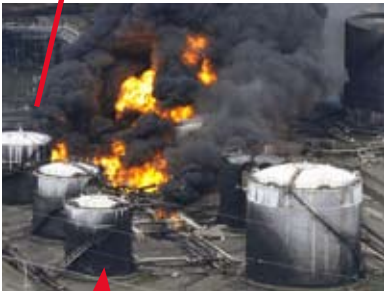
View of the road/rail loading station during the fire (amateur photos). A leak on a petrol pipe is the likely cause of the hydrocarbon vapour cloud, which ignited
