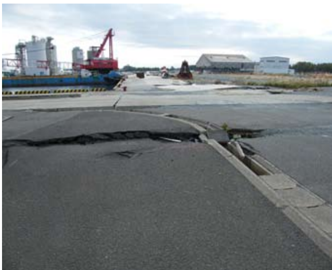
Subsidence of the docks near the Port of Soma concrete plant (Source : DGPR)
