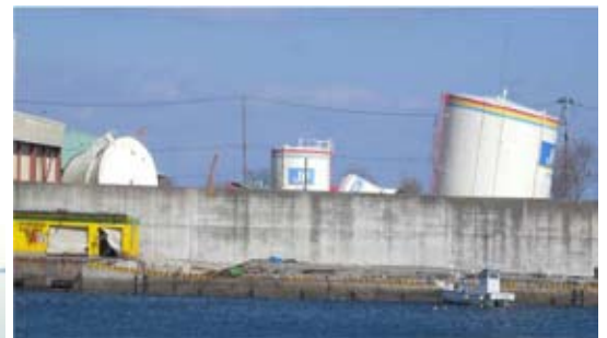
Storage tanks displaced after being submerged (4.3 m) in the Kuji oil terminal (amateur photo)
