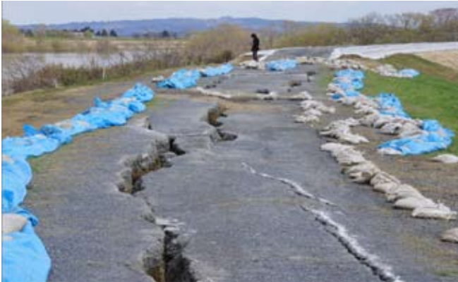
Cracks on a dike on the Naruse river (Source : EERI)
