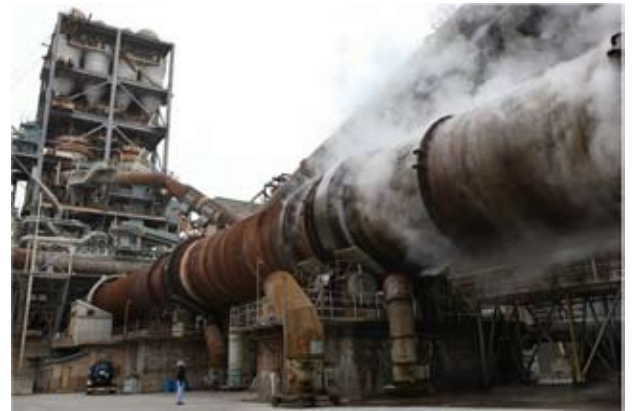
The elevated rotary kiln, spared by the tsunami, being brought back online (Source : Taiheiyo cement)
