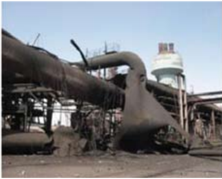
Damage to a coke oven gas pipe (Source : Sumitomo)
