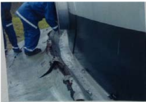
Storage tank foundation buckled by liquefaction in the Niigata oil terminal (Source : NRFID)
