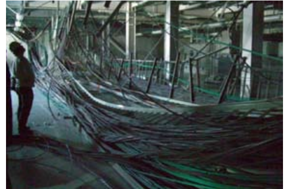
Collapsed overhead cable trays (Source : Renesas)
