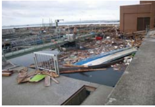
Debris in a settling basin at the treatment plant in the Port of Ishinomaki (Source : GWIA)
