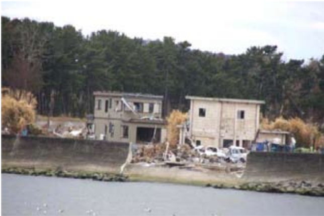
A dike section breached by the tsunami near the mouth of the Naruse river (Source : GEER)
