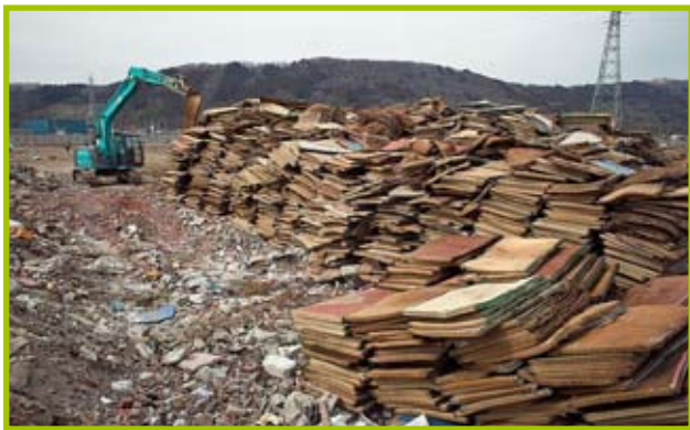
Combustible waste being stacked by category. Before being incinerated, these tatami mats were left out in the open air for several months to allow the salt in them to be naturally flushed out by rain (amateur photo)
