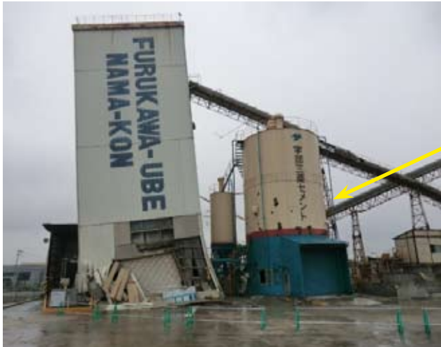
Seismic damage at a concrete plant in Ube (Source : Google Maps / amateur photo)
