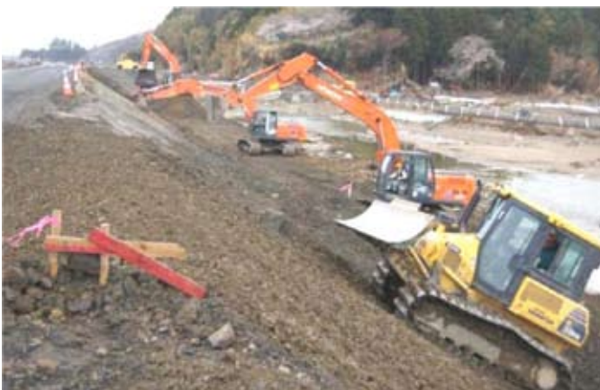
Dike along the Kitakami river being rebuilt in April 2011 after sustaining damage from the tsunami. The tsunami submerged the river's dikes along a distance of 5.5 km from its mouth and caused it to overflow its banks by more than 49 km inland (Source : GEER)
