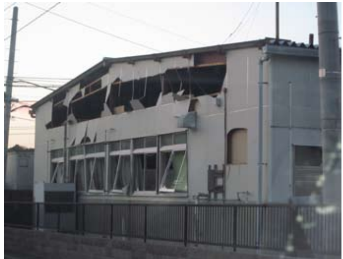
Effect of the KUREHA plant's hydrogen explosion on a neighboring building (amateur photo)
