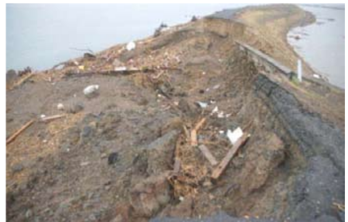
This dike section, located 4 km from the mouth of the Kitakami river, was heavily eroded after being submerged by more than 1.7 m of water from the tsunami (Source : GEER)
