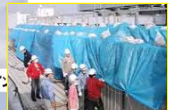
Workers scrambled to cover the roof the clean room with tarpaulins and sandbags to reduce contamination by outside air (Source : Renesas)
