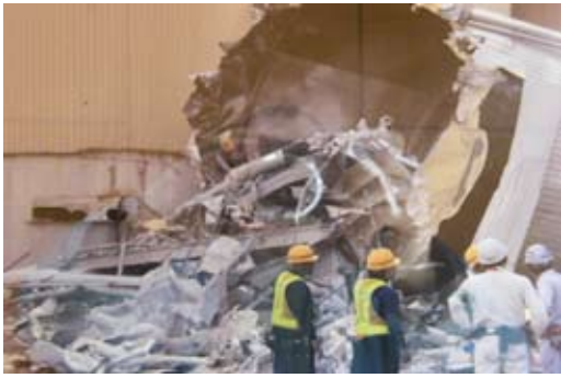
Damage sustained by one of the silos (Source : Kirin)
