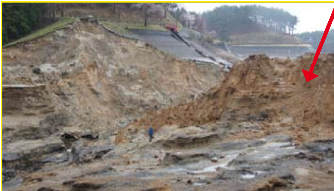
Breach in the main dam (Source : GEER / L.F HARDER)
