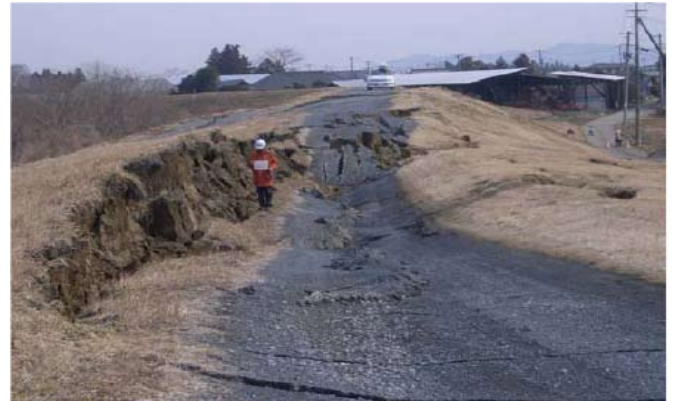
More than 2 m of settlement from vertical liquefaction were measured on this portion of the dike (Source : MLIT)
