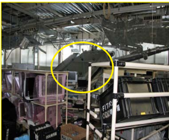
This air conditioner collapsed onto the spare parts racks on the second floor (Source : Fujitsu)
