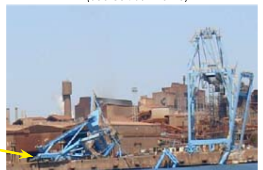
Damage to the sinter conveyor (Source : Sumitomo)
