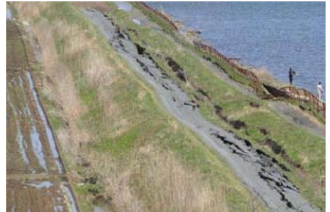
Liquefaction along the right bank of the Hinuma river (Source : GEER)
