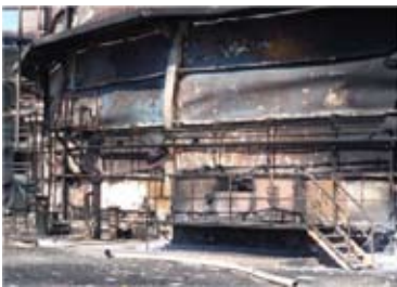
Top and base of the gas holder after the fire (above) and after being repaired in April 2011 (below)
