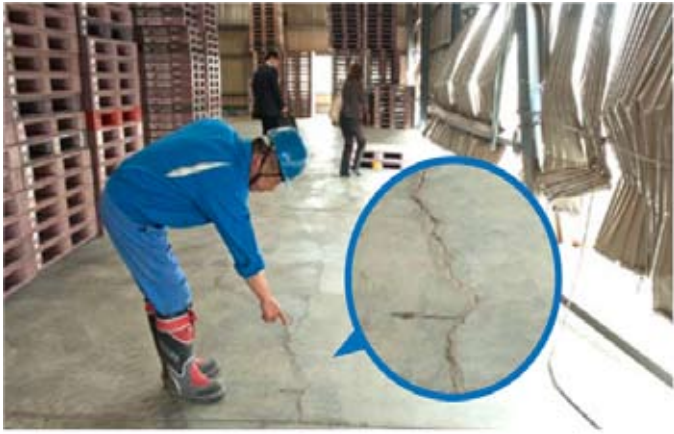
Floor cracks caused by liquefaction (Source : JPR)
