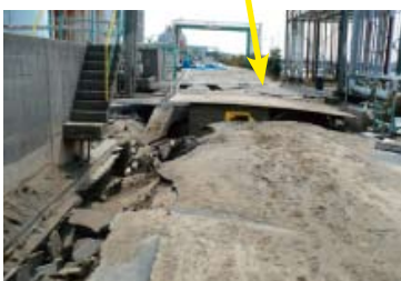
Road liquefaction between two production units (Source : Asahi glass )
