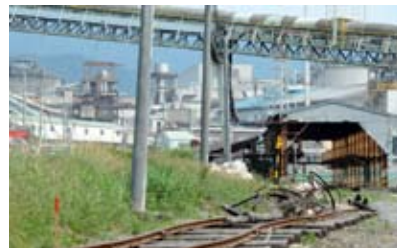
The tanks used to store fuel oil (supplying the rotary kilns) and bulk raw materials storage areas (clay, silica, etc.) were swept away by the tsunami
