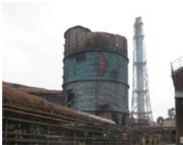
Top and base of the gas holder after the fire (above) and after being repaired in April 2011 (below)
