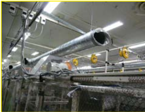
Failure of the duct used to supply the server ageing test equipment (Source : Fujitsu)
