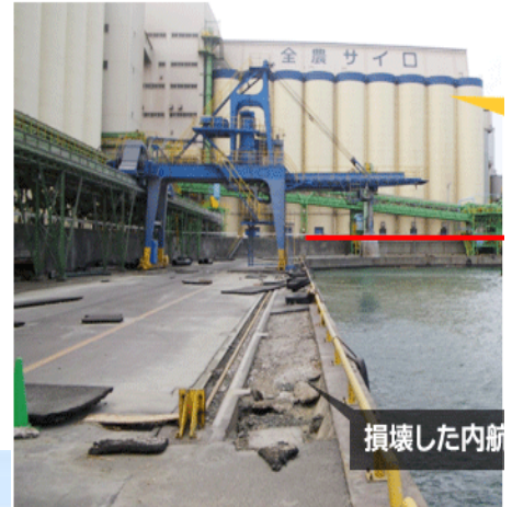
Above: exterior and interior photos of a grain silo damaged by the tsunami and its debris near Natori (Source : DGPR), Right: liquefaction of the dock of a grain silo in the Port of Kashima (source: METI)
