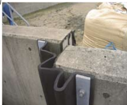
Bund walls buckled by liquefaction in the Kashima oil terminal (Source : NRFID)
