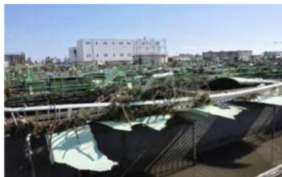
External damage: aeration tanks, pipes, treatment equipment (Source : Miyagi Prefecture - JWSA)
