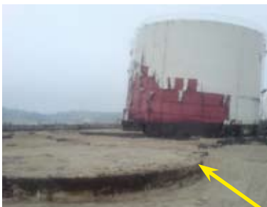
Fuel-oil storage tank pushed off its foundation by the tsunami (amateur photo)
