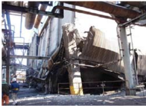
Damage to the base of the coke oven (Source : Sumitomo)
