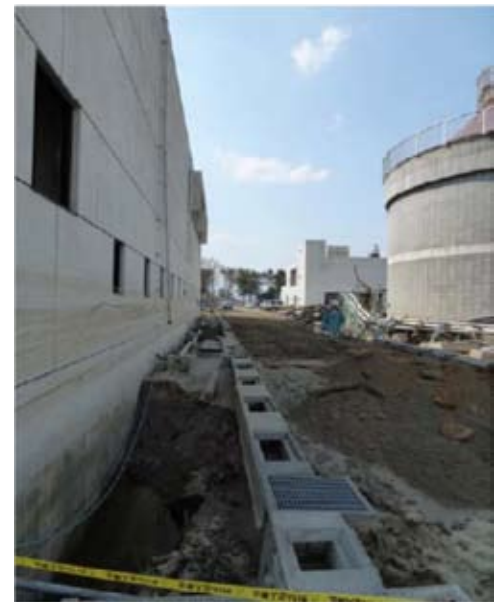
Soil erosion from the tsunami in a WWTP (Source : Miyagi Prefecture)
