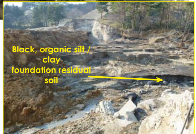
View of the foundation of the main dam following the breach (Source : JCOLD)
