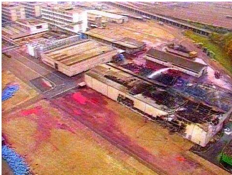
Figure 2 – Overall view: burned warehouse and pink firefighting water http://www.wissen.swr.de/sf/begleit/bg0016/nm15h.htm
