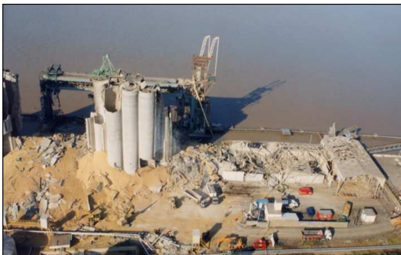
Northern silo zone
