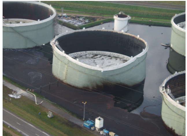
Figure 1 shows a picture of the situation in the bund the morning after the major accident happened.
