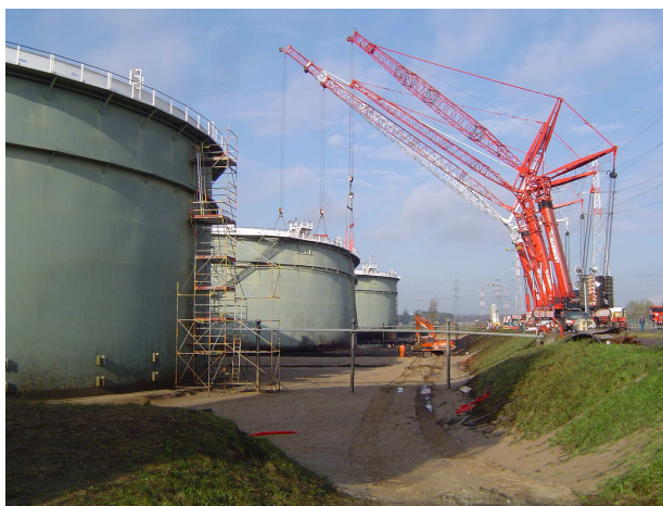
Figure 4: Major cranes stabilising tank D2
